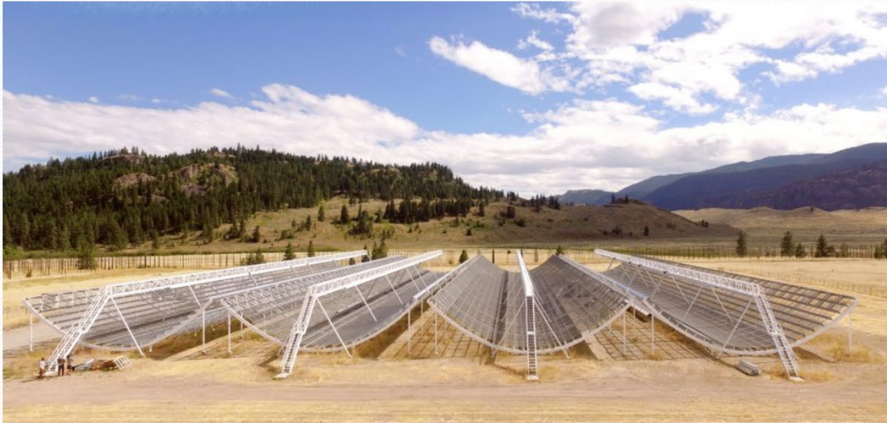
CHIME's huge reflectors are 100m long and each one measures 20m across. (Credit: CHIME)
