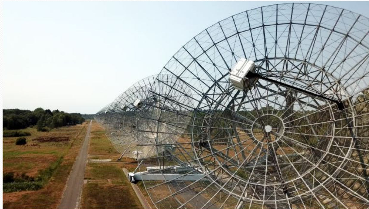
The upgrade means that the Westerbork Synthesis Radio Telescope can now map a patch of the sky 37 times the area of the full Moon. (Credit: ASTRON)
