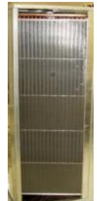
Water Coil (One of two)
