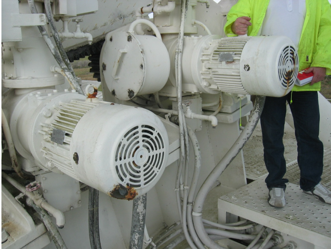
Elevation motor assembly – April 2009
