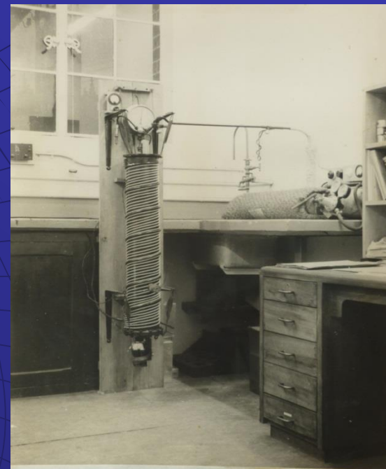
Plate 4. The Ionization Chamber and Gas Filling Line.
